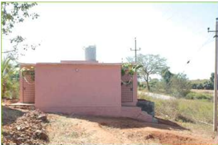
Healthy schools initiative - toilet blocks interior, exterior
