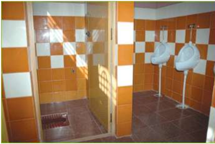
Healthy schools initiative - toilet blocks interior
